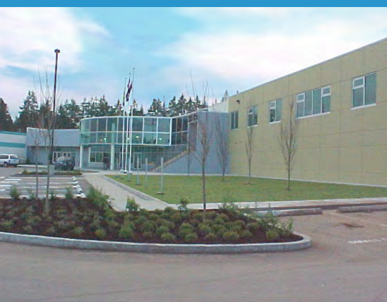
Oceanside Place Multiplex Arena
