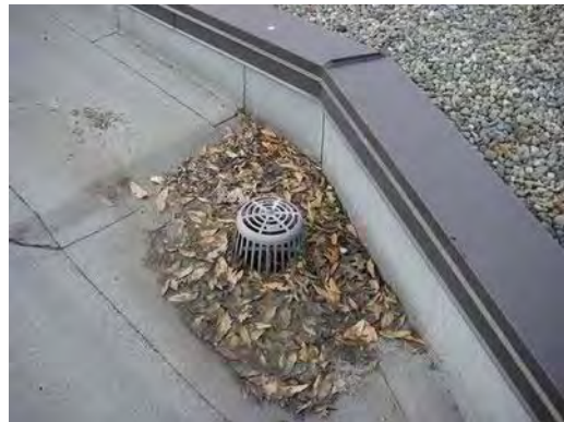
PLUGGED ROOF DRAIN
