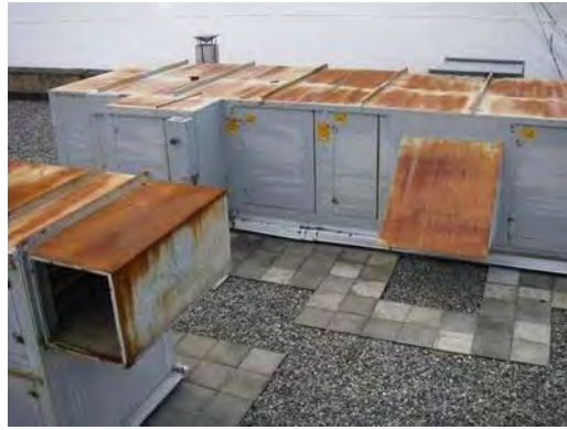
CORRODED HOUSING
