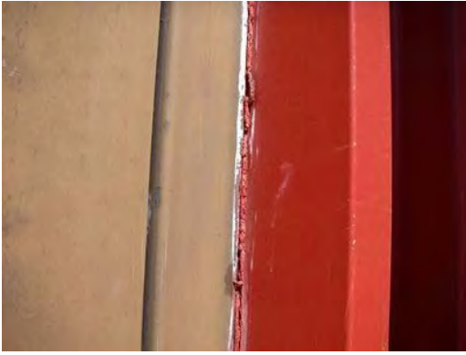
SEALANT FAILURE
