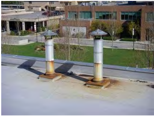
CORRODED B-VENTS
