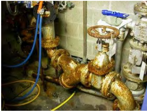
CORRODED PIPING
