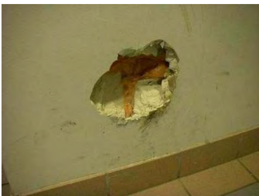
DRYWALL DAMAGED
