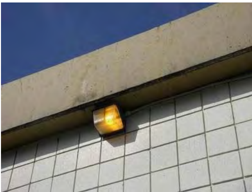
FAULTY TIMER/PHOTOCELL
